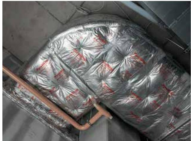
This scrim provides additional handling strength in addition to providing protection against moisture absorption.
